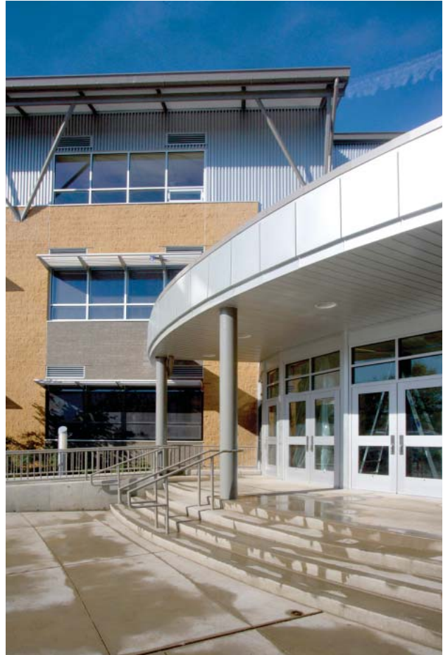
Photo courtesy of Graham Contracting
