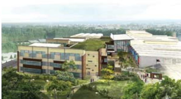
Denny International School is co-located with Chief Sealth High School. A light filled galleria joins the two campuses. (Images courtesy of DKA)
